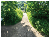
Shale ramp leading up from river – FINISH POINT
